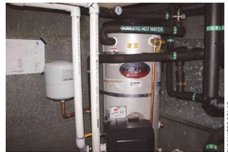
The Erkelens' smallest array, with four Schüco collectors and a single Phoenix storage tank, supplies nine apartments in an older building.
